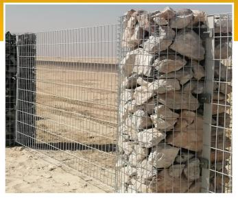
300x70x6 mm Welded to the steel post The fence panel will be fixed to it by 10mm bolts and nuts
